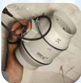
Carry out the wiring connections
