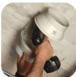
Fix the support bracket
