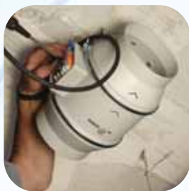
Carry out the wiring connections
